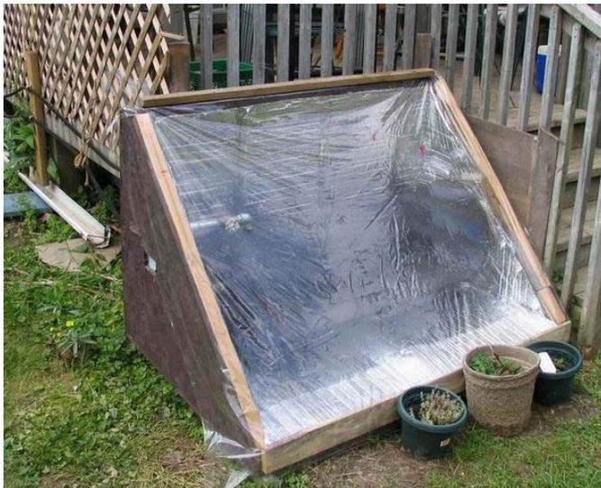
Once water was flowing from this valve it was closed and the inlet valve opened. The loop through the solar collector was now complete and ready to feed into the gas fired tank. The cut off valve in the original line was closed and we then had water flowing through the solar collector and pre-heating before it went into the gas fired hot water tank. The plastic aperture cover was put into place. My unit uses a
