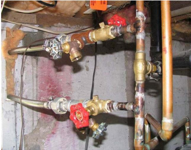
were checked here. We had to tighten some of these to stop minor seepage. Remember that you must use thread sealer, either plumbers stick or sealing tape, on these threads. Once water began to come out of the bleeder on the tank, that valve was closed. The next step was to open the boiler drain on the hot water feed line near the gas fired tank, allowing the air to escape from the line and water to flow down from the solar tank.
